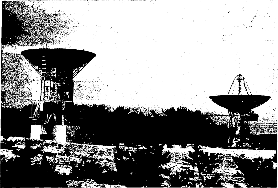
Figure VI-3—Transmitting site at Kashima (10-meter transmitting antenna at left; 30-meter receiving antenna at right).
